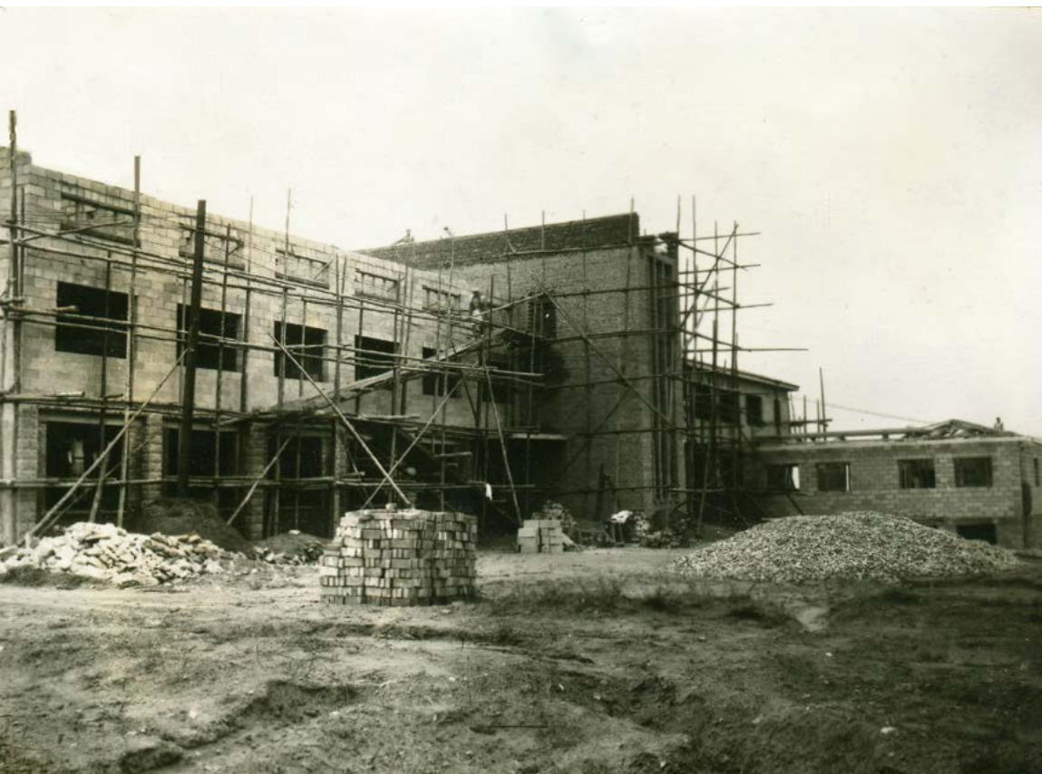
The Novitiate House Under Construction
