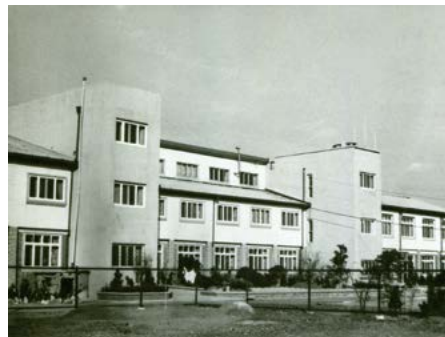
The building completed, view from south
