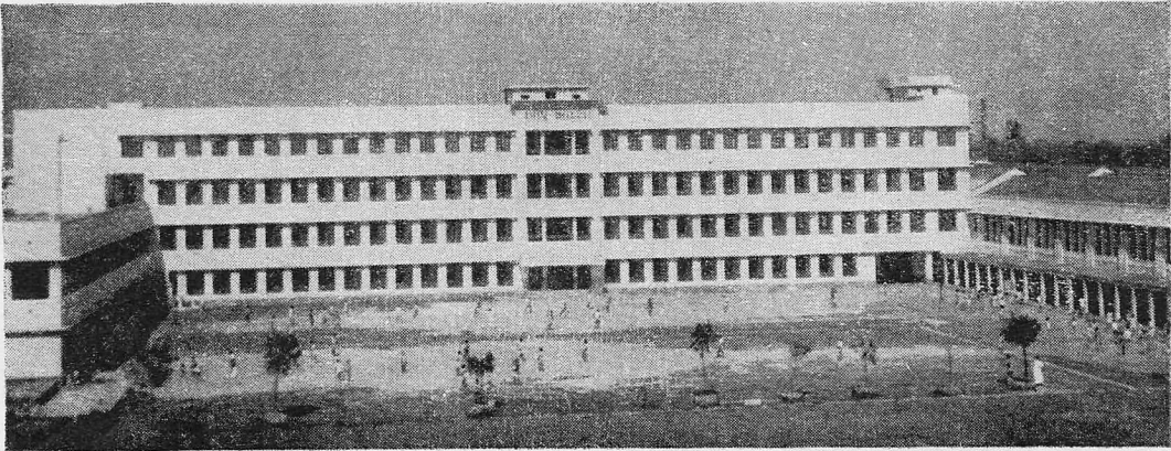
General view of the School Buildings
