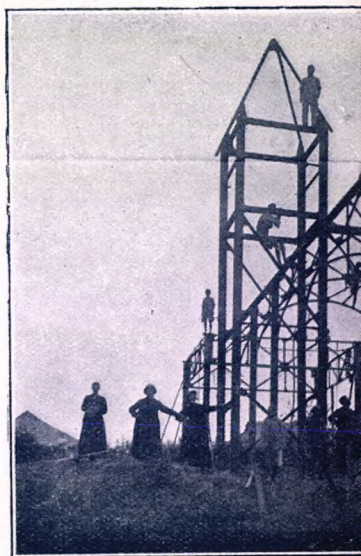
Shillong (Assam) - Ossatura in ferro
